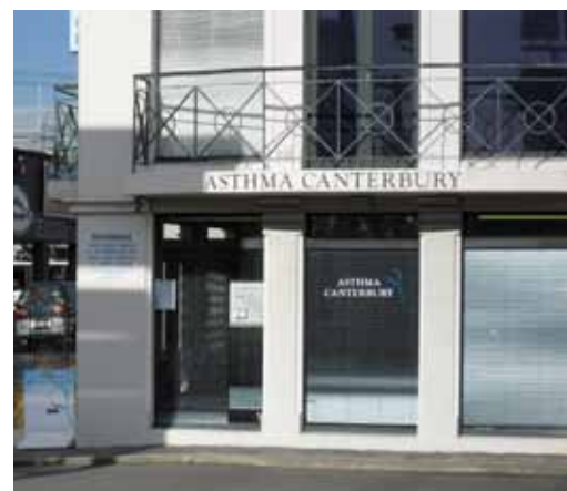
The Asthma Canterbury buildings in Christchurch were not badly damaged by the Canterbury earthquake of 4 September.
